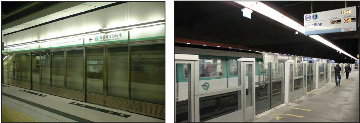
Figure 10. Platform Screen Doors and Platform Markings in Hong Kong (Left) and Paris (Right)
