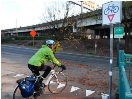
Figure 6.3 Yield Marking and Signage Connecting Two Bicycle Grade-Separated Paths in Portland (Source: http://bikeportland.org/2008/11/24/new-markings-meant-to-tame-bike-traffic-11270 )
