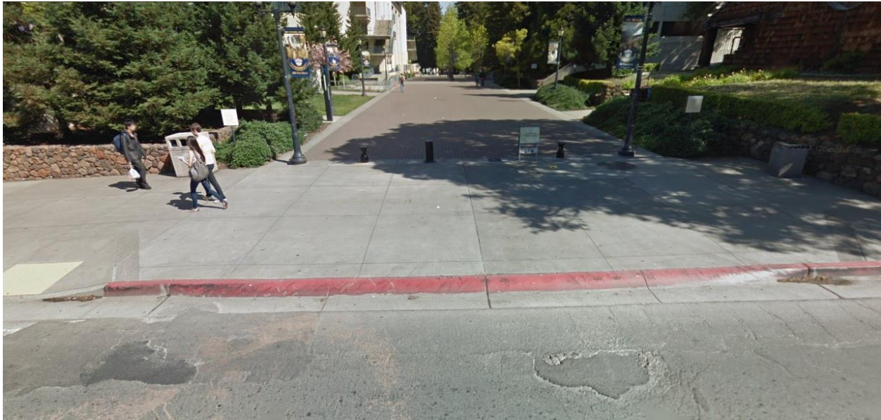
Figure 6.13 Rolled Curb along the Spieker Plaza Sidewalk to Facilitate Vehicle Access
